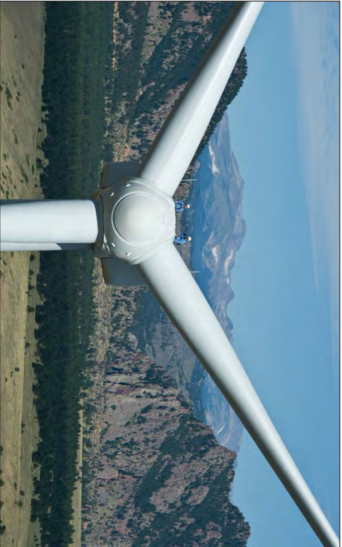
Activity 3 - 2500 - Aerial view of a techs working on the ALSTOM ECO 100, 3MW horizontal-axis upwind turbine at NREL's National Wind Technology Center (NWTC). August 7, 2012. National Wind Technology Center, Colorado. (Dennis Schroeder/NREL 21869)
