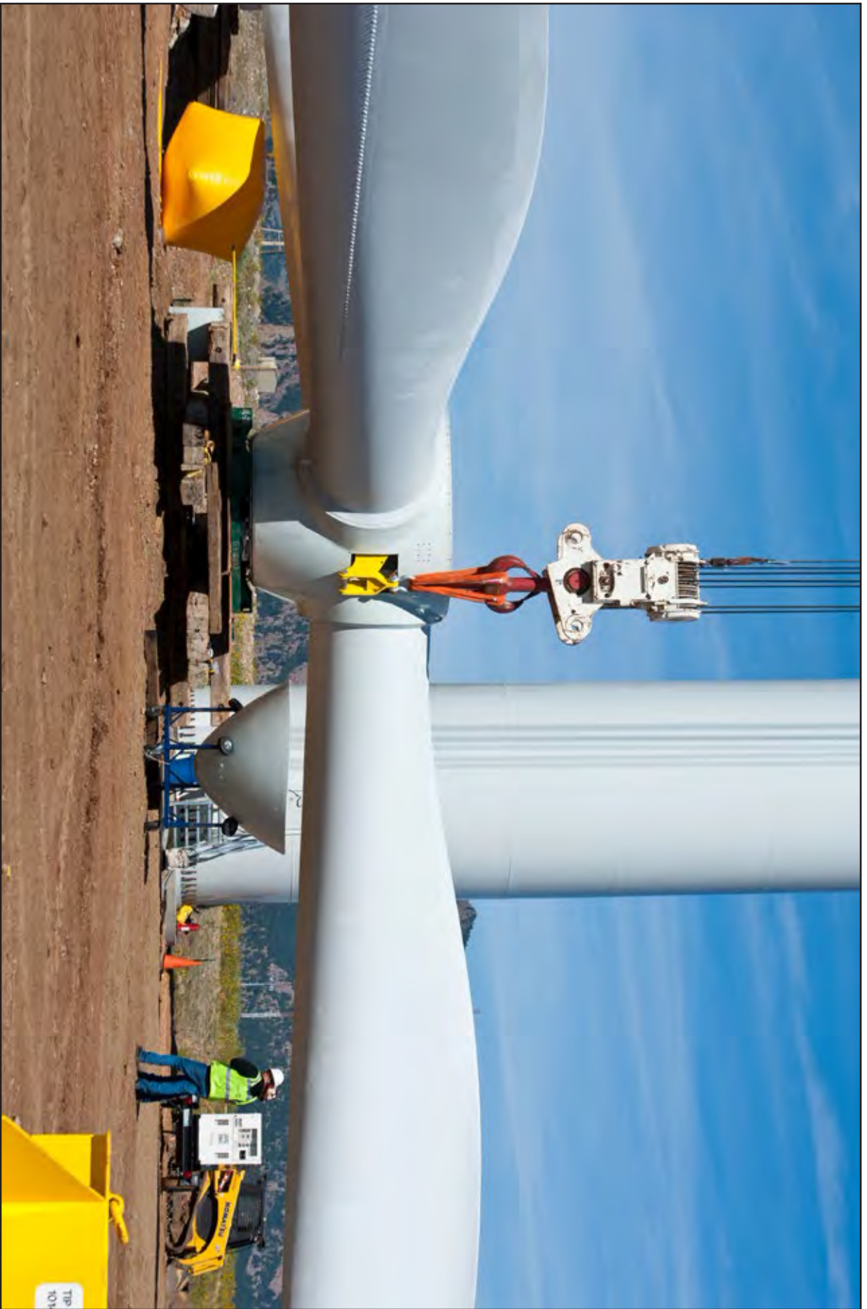
Activity 3 - 2555 - Workers use a giant crane for lifting the blade assembly as work continues on the 2 MW Gamesa wind turbine being installed at NREL's National Wind Technology Center (NWTCC). September 22, 2011. National Wind Technology Center, Colorado. (Dennis Schroeder/NREL 20869)
