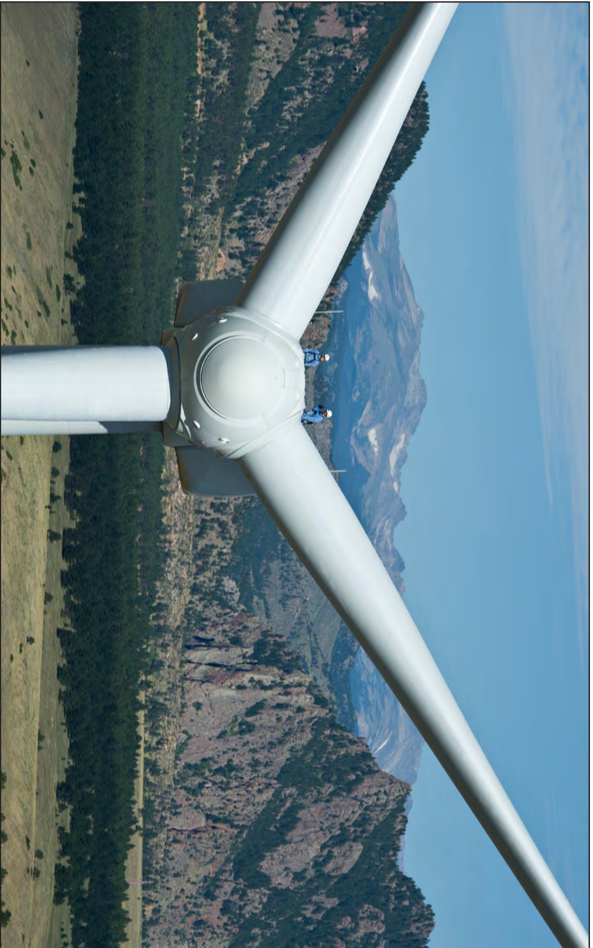
Activity 3 - 2500 - Aerial view of a techs working on the ALSTOM ECO 100, 3MW horizontal-axis upwind turbine at NREL's National Wind Technology Center (NWTCC). August 7, 2012. National Wind Technology Center, Colorado. (Dennis Schroeder/NREL 21869)
