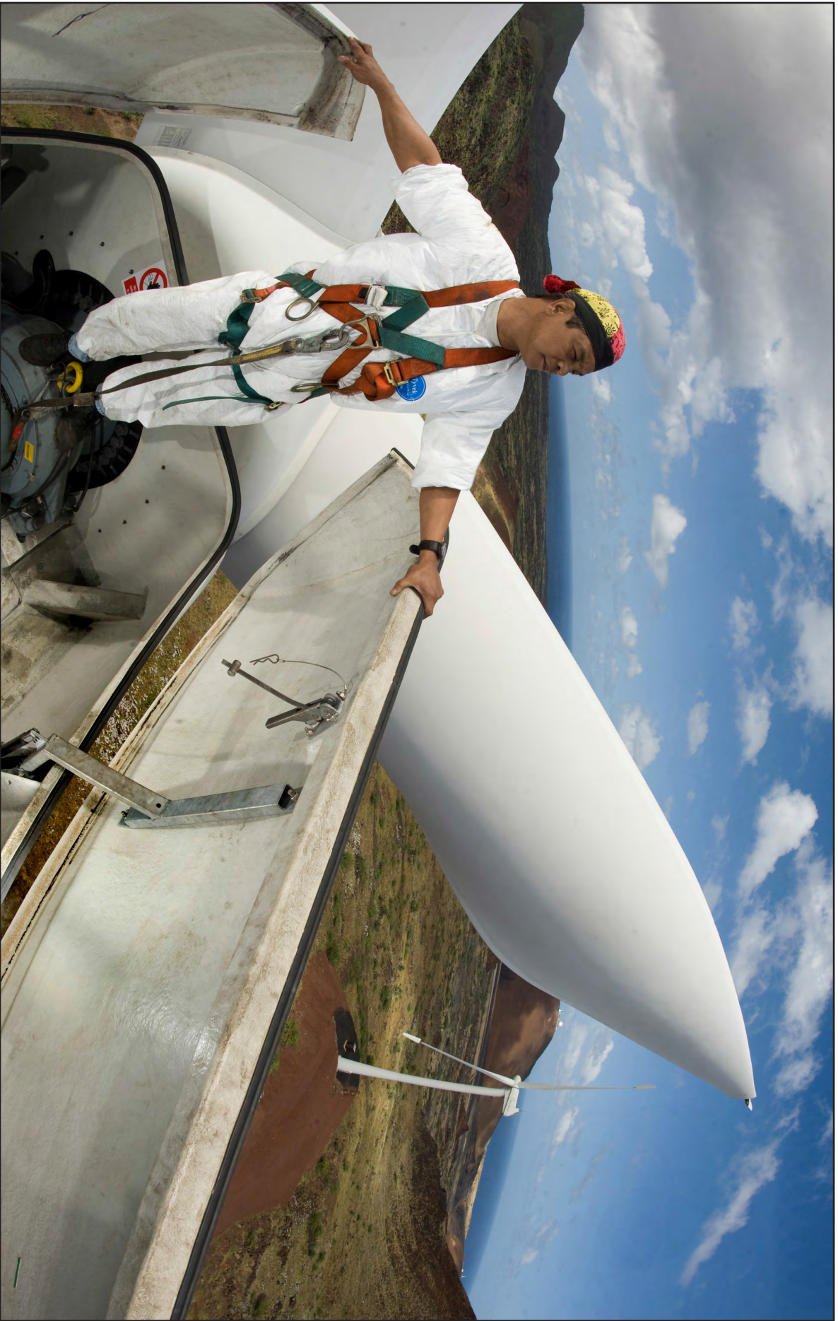
Activity 3 - 2599 - Damien Cuello uses the more than 110-foot high view from a 900kW wind turbine to get a better visual inspection of the other 900kW turbine and four other 225kW turbines at 45th Operations Group Detachment 2, Ascension Auxiliary Airfield, South Atlantic Ocean. The power house operator/mechanical associate is tethered and stands on the drive-line to get parallel views of the other generator housings. Cuello is a Computer Sciences Roytheon contract associate in charge of maintenance for the 6-wind turbine facility. June 24, 2009. Ascension Island. (Lance Cheung/U.S. Air Force)
