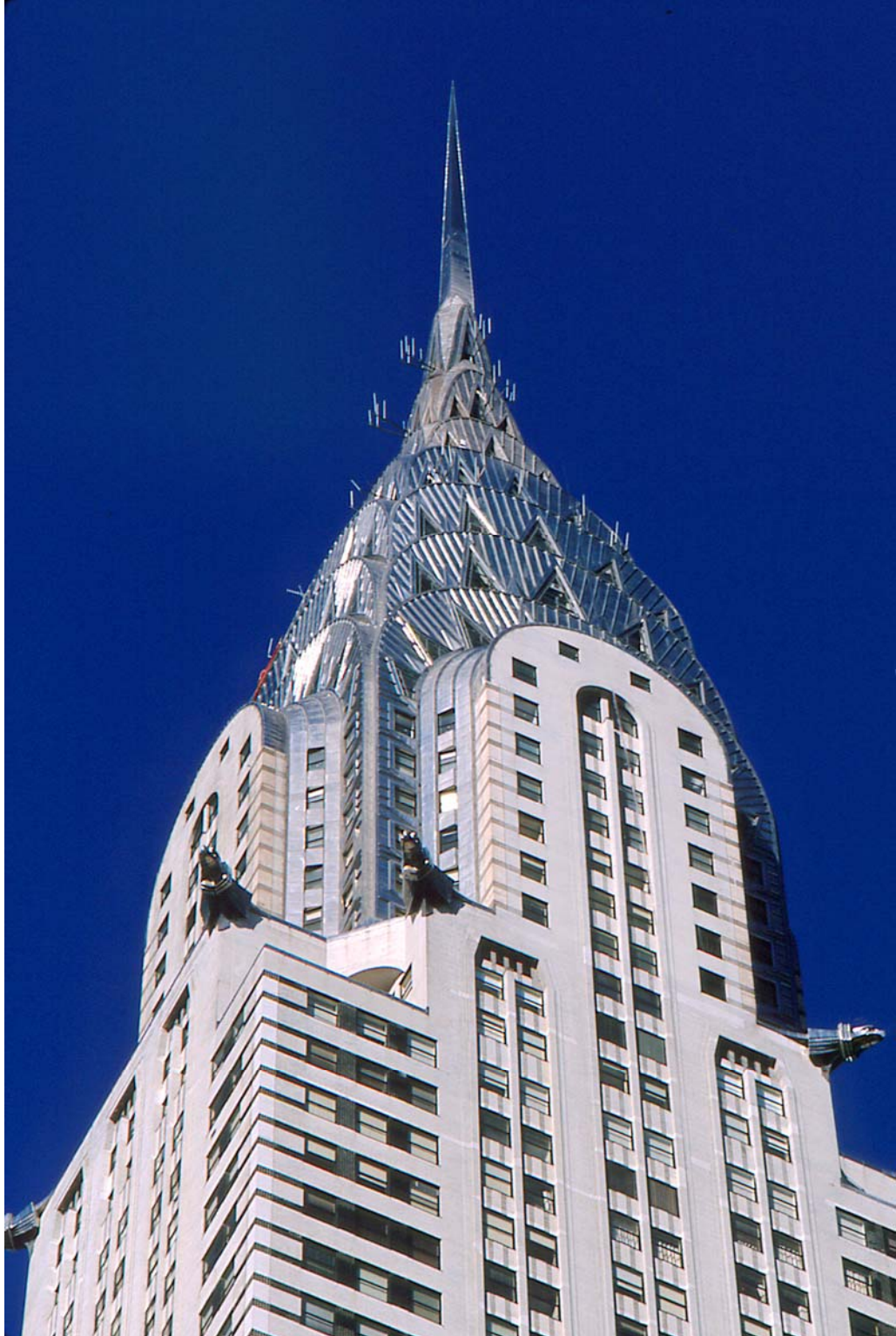
Figure 8. William van Alen (American, 1882/3-1954); Chrysler Building ; steel frame, brick, concrete, masonry, and metal cladding; 1928-1930; H: 1,046 ft. (318.8 m.); 42 nd Street and Lexington Avenue, New York, NY. Photograph © Alan Schein Photography/Corbis.
