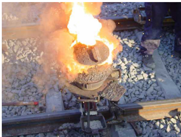
Figure 7-9. Thermite Welding
