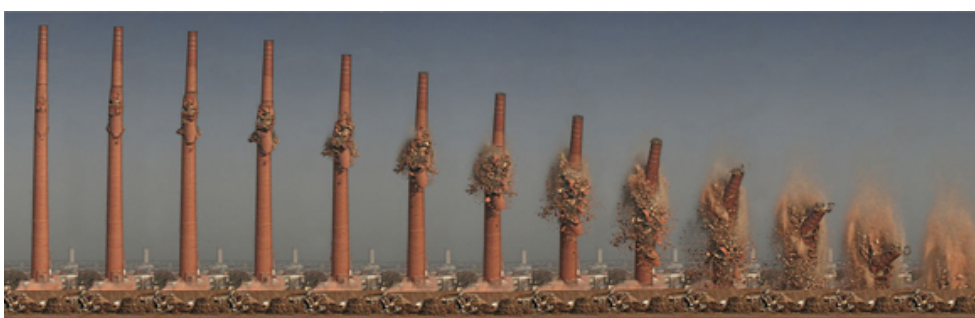
High explosives, like the one used in the demolition shown above, release tremendous amounts of enthalpy very quickly due to the formation of high-enthalpy bonds. This, in turn, heats the air and the reactants, which then rapidly expand causing destruction. © Wikimedia Commons, Creative Commons License 3.0. Author: Heptagon, 2 December 2006.
