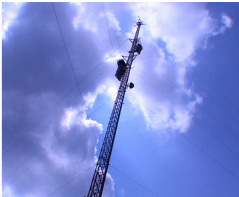
Figure 16. Tall tower monitoring station for atmospheric sampling
