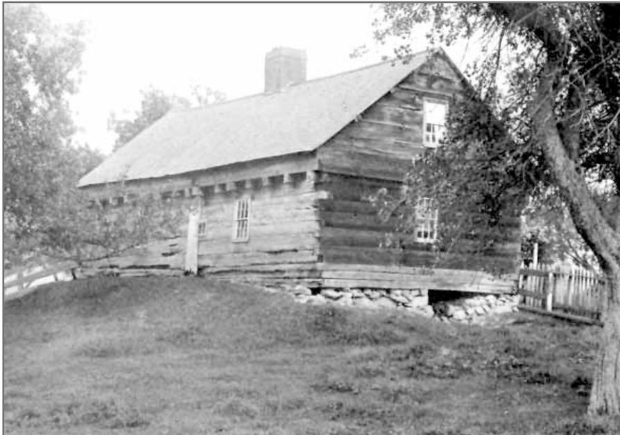
House built before 1698. Such houses are called garrison houses and were sturdily built to act as fortresses. Although the roof is new and the glass in the windows is probably modern, the chimney may be the original. Brickyards were among the first enterprises started in the Massachusetts Bay Colony.
