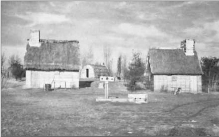
One room cottages built by the Puritans in their early years. Note that the chimneys are made of stone, clay, and wood and that the only visible windows are covered with wooden shutters.
